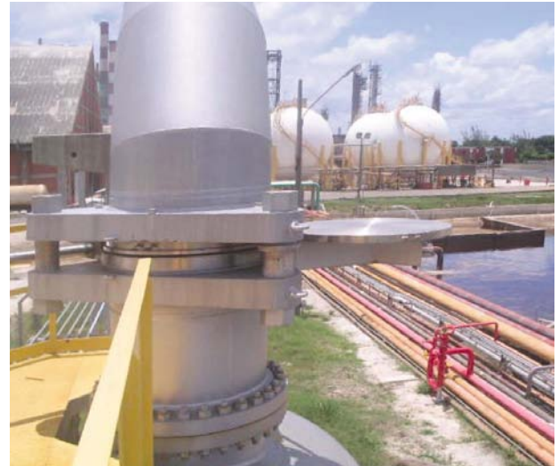
Cam-Set® DN 500 (20"), ASME 150# with spectacle plate support
